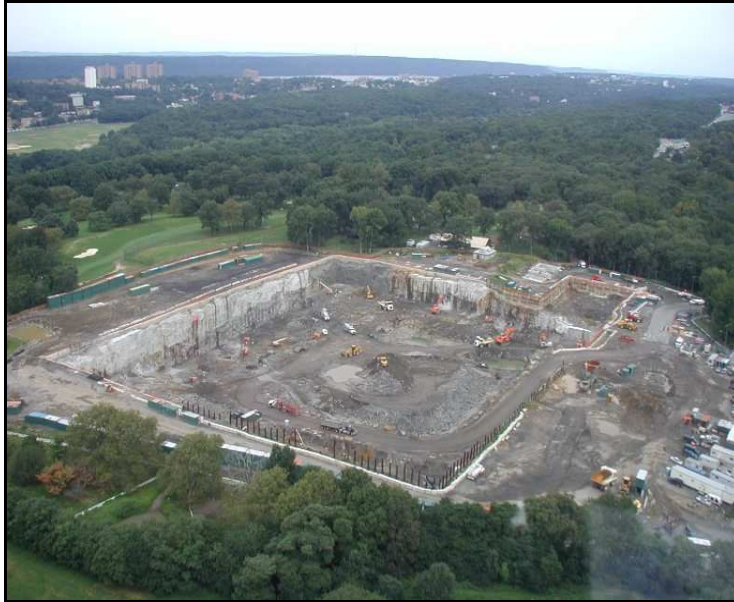
Figure 1. Croton Water Treatment Project in the Bronx, New York
